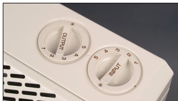
The **Input control dial**, which should be on the *right hand side*, controls how much the heaters charge-up overnight and during the afternoon, with `5/6' being the highest setting.
