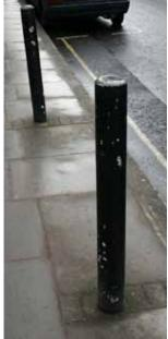
Multiple signs on listed lamp posts and bollards made from pipe filled with concrete
