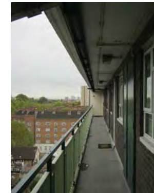
Tollgate House Existing Gallery Access with Metal Balustrading
