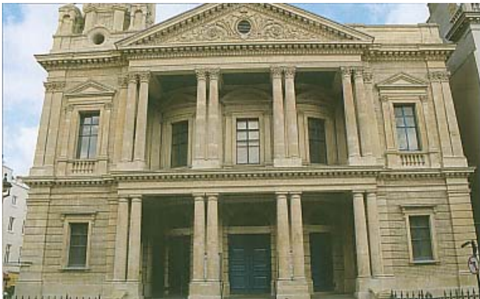
Hinde Street Methodist Church, W1, 1881-7 by James Weir, listed Grade II. Front elevation, built in limestone and white brick, after cleaning and repair. All the repairs have been carried out by piecing in matching stone to heavily eroded areas. Stainless steel wires have been installed on ledges to deter pigeon roosting.
