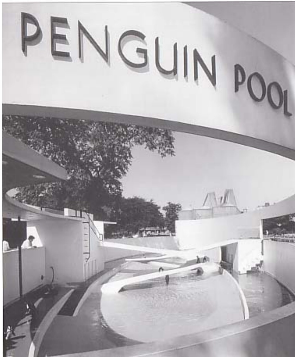
The Penguin Pool, London Zoo. Grade I listed structure dating from 1934 designed by Lubetkin and Tecton. Reinforced concrete structure with cantilevered interlocking spiral ramps. The repair of the pool has had to balance the need to improve weathering details while retaining the purity of the original design. Special provision has been made for future planned maintenance.
