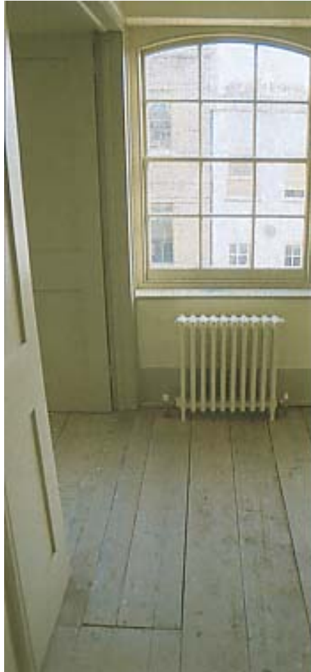
Wide timber floorboards (68 Dean Street, Soho)
