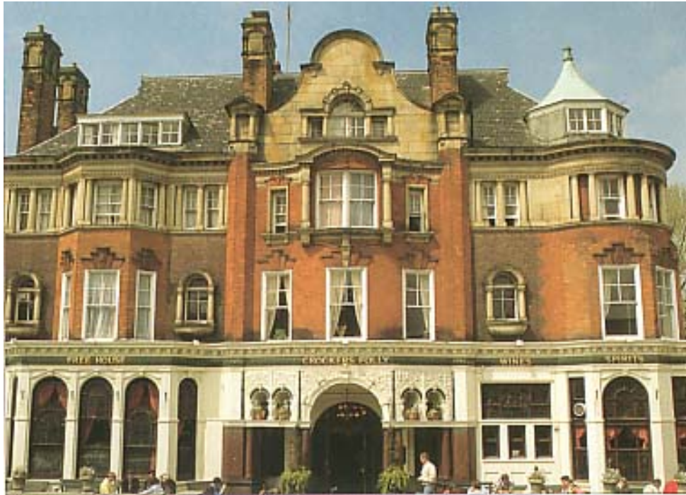
Crockers Folly Public House, Aberdeen Place, NW8. A lavishly constructed pub dating from c.1900, which retains a fine interior with original fittings. Listed Grade II*.
