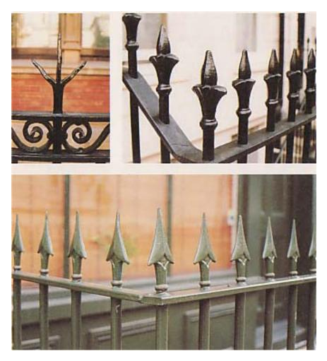
Wrought iron, cast iron and mild steel. Examples of wrought iron (top left), cast iron (top right) and mild steel (bottom) finials. Note the smooth texture and hand made quality of the wrought iron head, the rough texture and robust form of cast iron and the mechanical uniformity and simplified assembly details of the mild steel panels.
