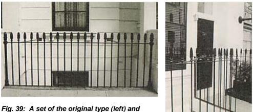
Fig. 39: A set of the original type (left) and (right) an incorrect reproduction
