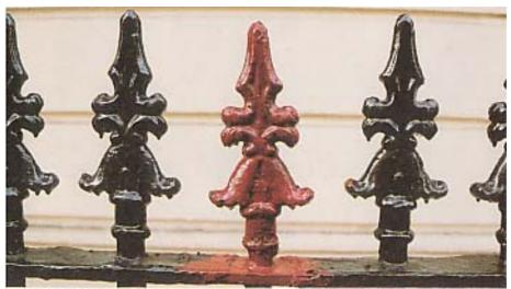
Treatment and protection of rust affected connection point. Note the complete removal of old paint before the application of the protective primer.
