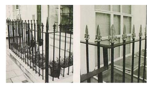
Examples of mild steel replacement railings: Where consent is required for the installation of mild steel railings, the City Council will seke to secure that not only the heads and finials but also the size of the bars, their spacing and all structural details are made to correct authentic design. On listed buildings, the City Council may require the use of the original type of metal. The above two examples are not entirely successful.
