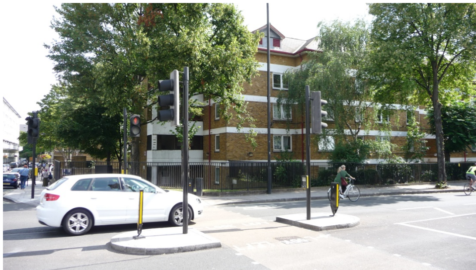
Penn House, looking east from Lisson Grove, with Lilestone Street on the left
