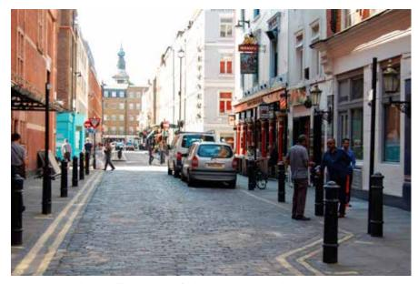
The eastern end of Romilly Street has flush kerbs and is paved with granite setts.
