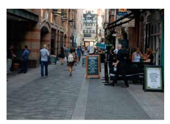
Kingly Street: resurfaced, raised carriageway and loading bays, paved with tricolour grey granite setts.
