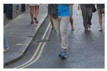
Typical condition: concrete paving with granite kerbstones and asphalt carriageway. Where footway widths are sufficient aim to maintain this material palette. In many cases better maintenance is required, however material changes are not recommended.
