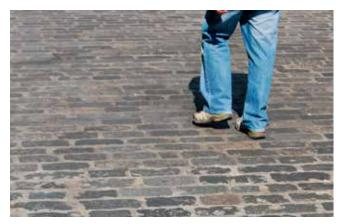
Paving for edge streets or pedestrian spaces should still feel like it belongs in Soho. Reclaimed granite setts laid flush have been successfully used on Rupert Street.
