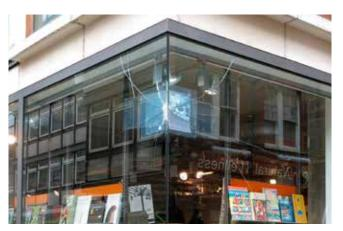
Facade damage caused by a delivery vehicle negotiating a tight corner.
