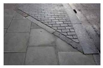
Potential improvements where footways are very narrow: concrete paving with granite kerbstones, raised parking/loading bays in dark, uniform granite setts, re-laid asphalt carriageway potentially level with footway if this is beneficial.
