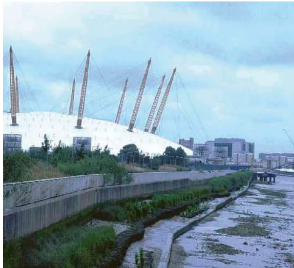
Terraces at the O 2 – cheaper to build, subsequently increased value of the land and enhanced local ecology
