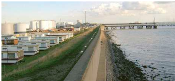
Flood defences at Canvey Island
