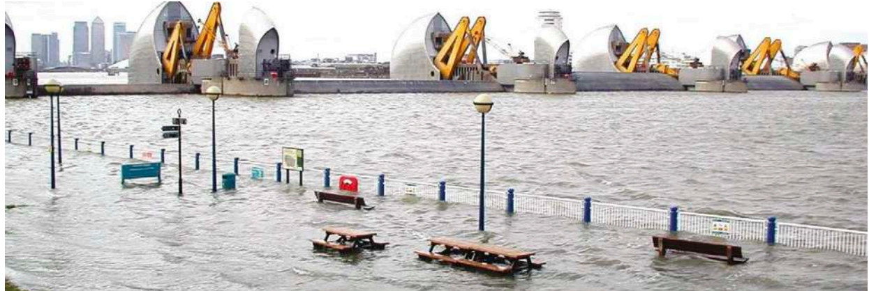
Surge tide event at the Thames Barrier
