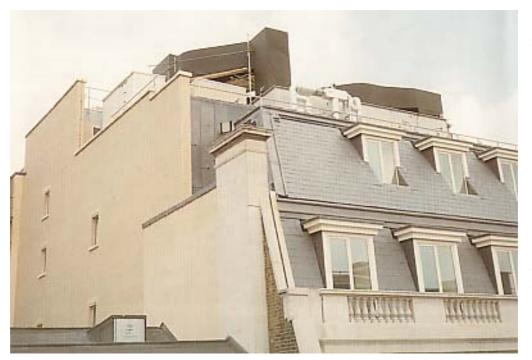
Air-conditioning plant should alwavs be located out of sight, within the envelope of the roof or screened by an appropriately designed roof-like enclosure. **Proposals for** new buildinas should make adequate provision for plant.
