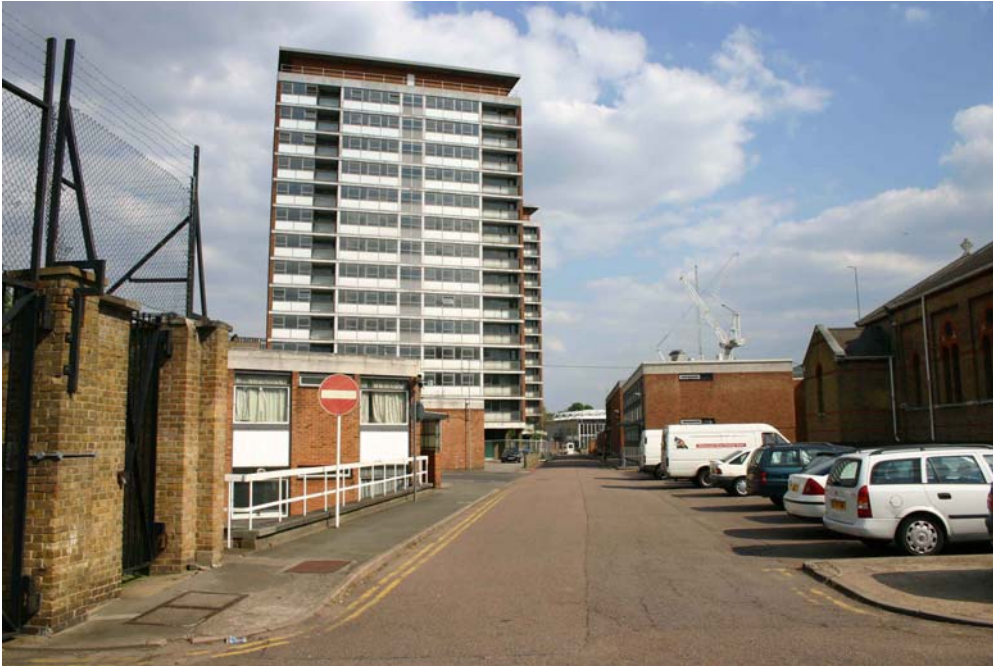
Barracks tower blocks from main internal road looking east
