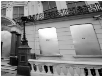
Vacant units are vacant residential properties returning to use
