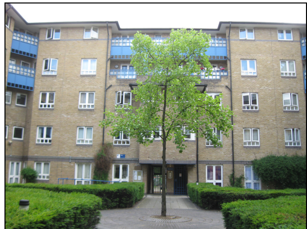
Phase One Lockbridge Court
