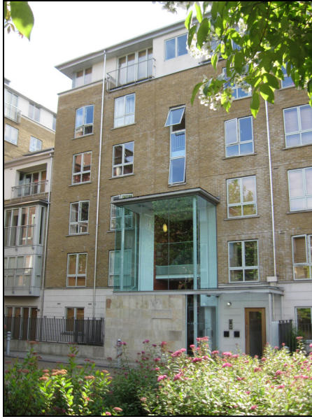
Phase Three Carlton Gate Elm Court
