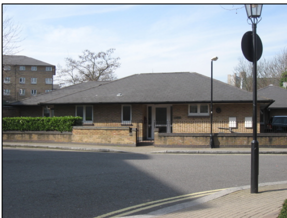
Front elevation of 1-2 Elmfield Way
