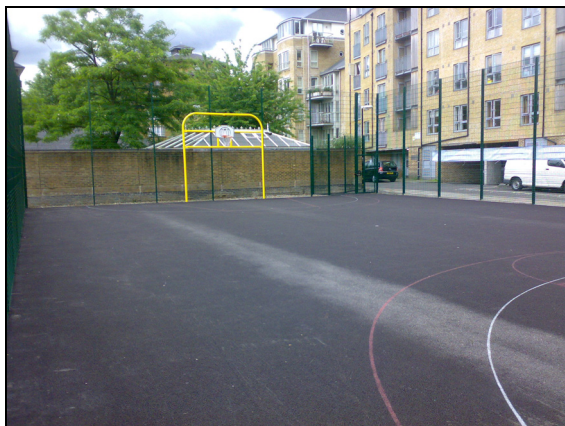
Inside MUGA on N3 Site
