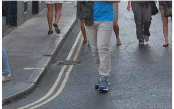
Typical condition: concrete paving with granite kerbstones and asphalt carriageway. Where footway widths are sufficient aim to maintain this material palette. In many cases better maintenance is required, however material changes are not recommended.
