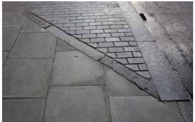
Potential improvements where footways are very narrow: concrete paving with granite kerbstones, raised parking/loading bays in dark, uniform granite setts, re-laid asphalt carriageway potentially level with footway if this is beneficial.
