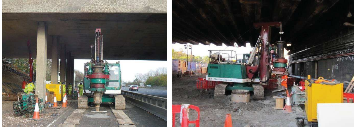
Figure 3: Martello Technique Piling
