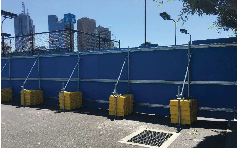
Figure 23: Example hoarding for Phase 2
