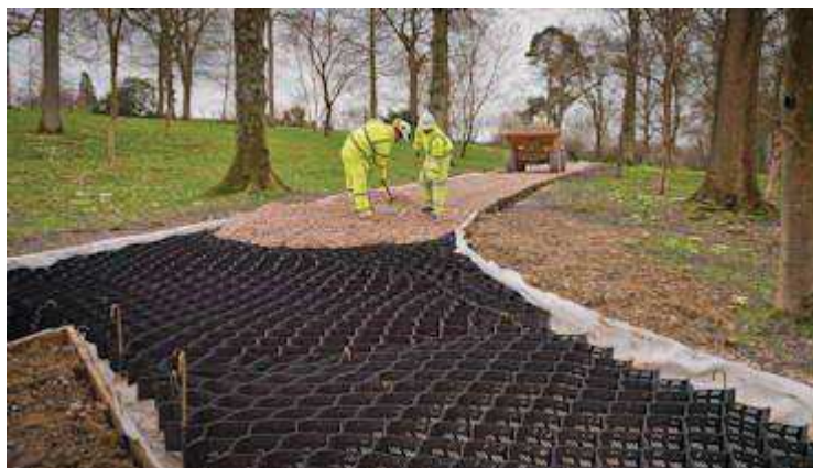
Figure 22: Indicative Cellweb Installation
