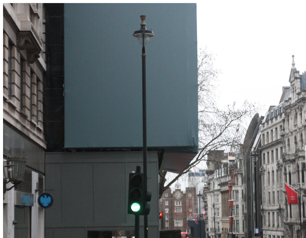
Image 46: Hoarding affecting the performance of column lighting
