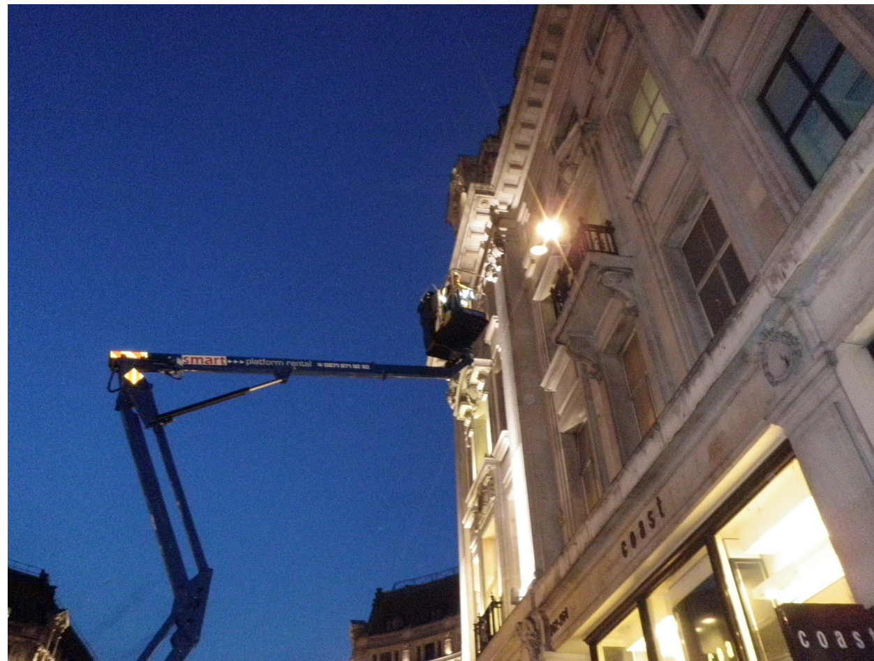
Image 49: Specialist tower wagon required to access wall mounted lighting
