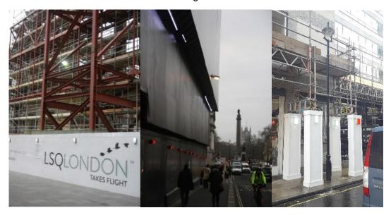
Temporary luminaires mounted on building support frame and poor practice where the existing column-based lighting is included within the scaffolding
