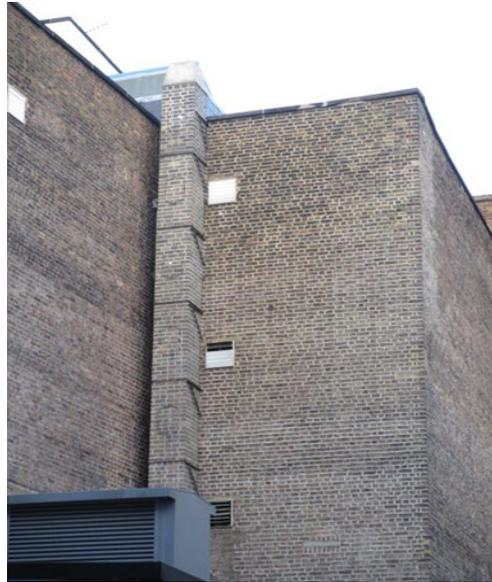
*Figure 2 Good aesthetic design of extract duct with matching pseudo brick effect (note includes access panels)*
