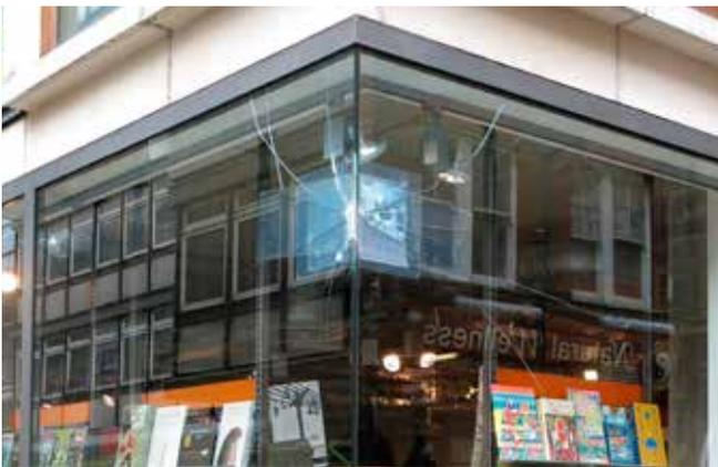
Facade damage caused by a delivery vehicle negotiating a tight corner.
