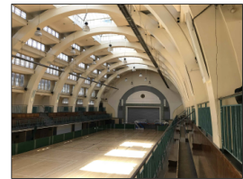
image of existing Sports Hall
