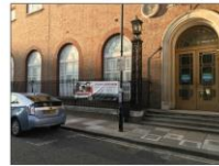
photo of proposed Marylebone Library entrance and new access ramp
