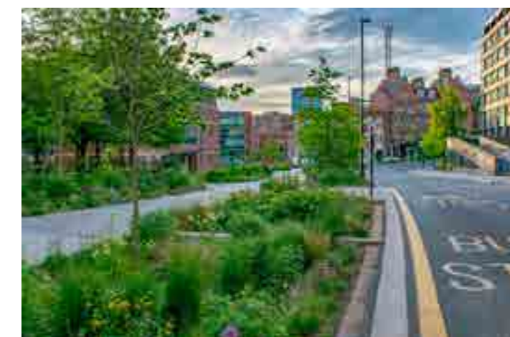
SuDS retrofit scheme - Grey to Green, Sheffield © Nigel Dunnett
