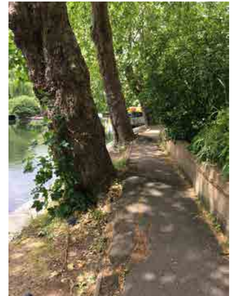
5. Uneven, narrow and inaccessible path along Rembrandt Gardens and the canal hinders on links to the water. Footway currently leads to dead end and lacks sufficient signage.
