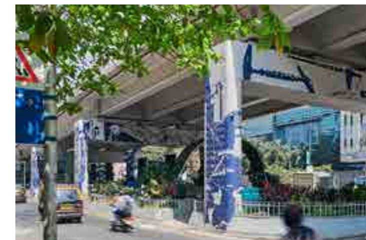
One Green Mile - Community space beneath flyover, Mumbai, by MDRDV & StudiPOD © Suleiman Merchant 2022.
