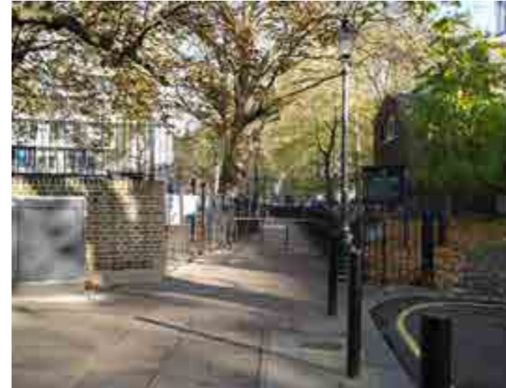
2. Church Yard walk is narrow. Railings at either cause obstruction and discourage accessibility. Channel-like feeling particularly in the evening and excess fences.
