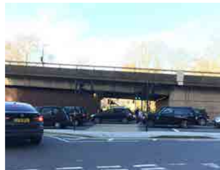
5. Hermitage Street at-grade crossing is key, but lacks complete infrastructure. The road layout forces you as a pedestrian to walk down the middle of Hermitage Street rather than into a footpath on either side
