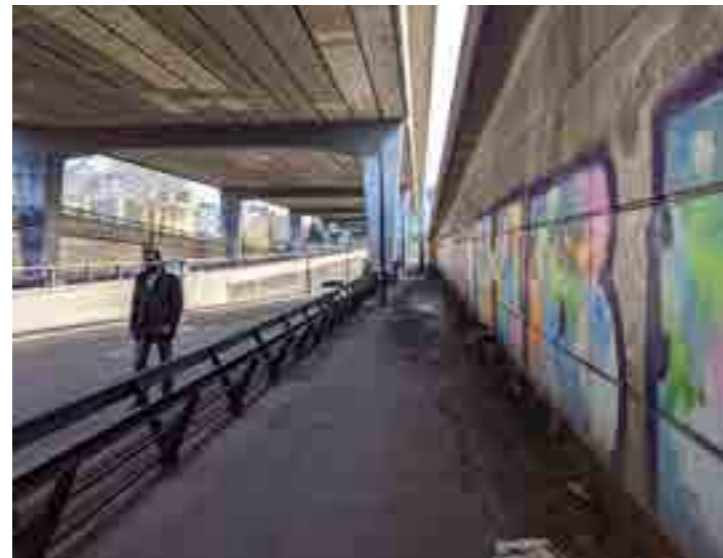
5. Route to Royal Oak Station is of very poor quality, noisy
