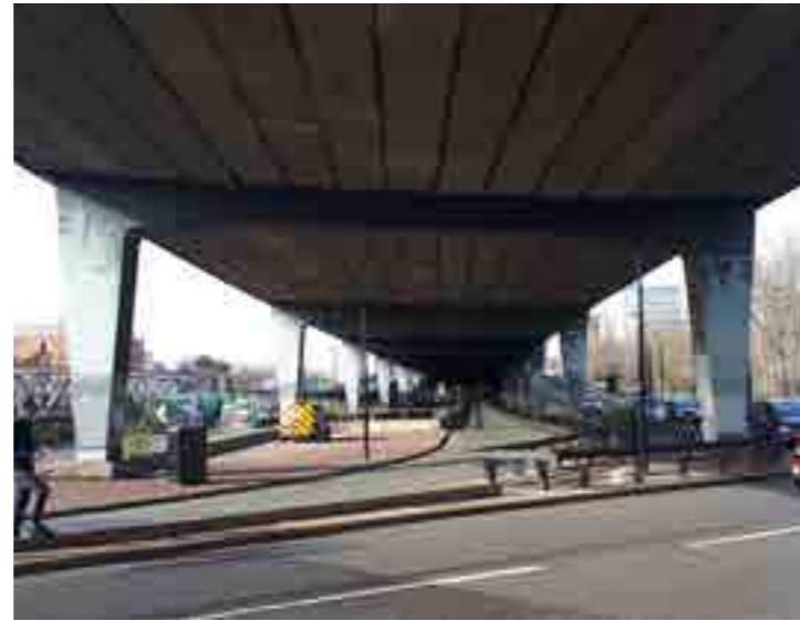
1. Underwhelming space under the Westway No crossing - convoluted routes for pedestrians
