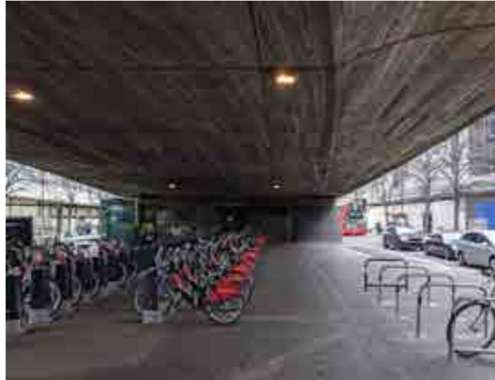
1. Existing Cycle Infrastructure beneath the Flyover
