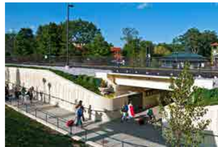
Safe & healthy underpass, Ravinia Festival Underpass, Highland Park, Illinois © SmithGroup
