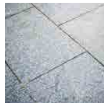
'Standard' surfacing e.g. Granite paving slabs
