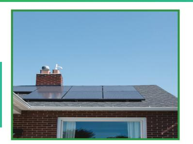
At this home, there are 10 solar panels installed on the roof. Together they will generate approximately 3300 kWh of electricity per year – enough to power the air source heat pump as well as the other electrics (lighting and appliances) in the home.
