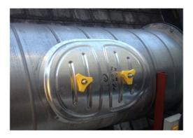
Figure 1 - Access panel for duct cleaning
