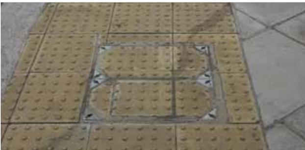
Tails to tactile paving at crossing and coloured slabs. Below: unremedied defects and cluttered junction design must be improved.
