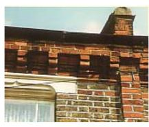
The projecting brickwork or corbellng below the eaves is very exposed to the elements. As a result the soft red bricks can become badly eroded.
