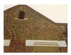
In this photograph the poorly applied pointing has overwhelmed the subtle textures of the brickwork. Compare with the more appropriate pointing between the window arches.
