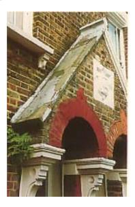
The original cantilever design of the porch canopy provided insufficient support for the weight, as a result of which structural defects to the wall and porch are common.
